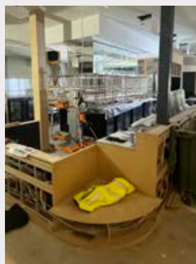
Above: Bar construction.
